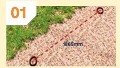
Mark the two post locations 1865 mm apart, centre to centre. This allows the 1.8m fence boards to slot into place when the posts are set.
