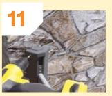
Using a 3mmdrill bit, drill two pilot holes into the post, using the two predefined holes on the cap as a guide.
