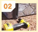
Fix the stopper to the wall post with two screws.
