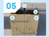
DO NOT over tighten the hidden fixing clip.
