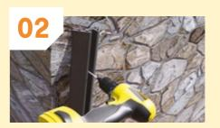
Level the wall post against the wall, keeping it straight and firmly on the ground. Using a 5mm masonry drill bit, drill 50mmpilot hole at the top into the wall.
