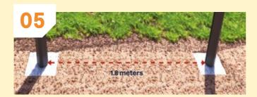
Place the second post and repeat, making sure the distance between posts stays 1.8m, recess edge to recess edge.
