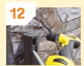
Fix the cap to the post with the supplied screws.
