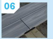
Where board ends meet allow an expansion gap (see expansion table) fit a second supporting noggin and fit a hidden fixing clip at the end of each board.
