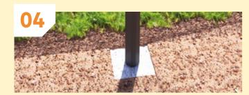
Following the manufacturer's guidelines, fill the hole with concrete, using supports and a spirit level to ensure it stays level on all sides.
