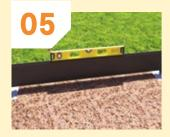
Using a spirit level, make sure the board is 100%level
