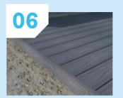
Use two colour coded screws at every joist.
