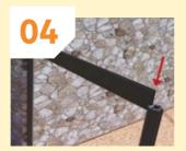
Insert the gravel board at the top of both posts and slide it down to the ground.
