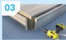
Skirt trims can be used to finish the deck. Fix with two screws at the recommended centres. Drill pilot holes before screwing.
