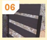
Slot in the first fencing board, ensuring it is level before adding the other boards. Each board should sit firmly on the last, similar to tongue and groove.
