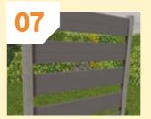
Once all fence post connectors are secured, slot 5 fencing boards in one by one, making sure each fits firmly on the bottom board, before stacking on the rest.
