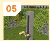
Next, fix the top of the fence post connector to the concrete post with the supplied screws.
