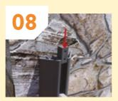
Slide a stopper onto each post to sit above the fence finishing rail.
