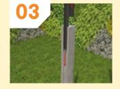
Insert the fence post connector into the concrete post recess and use a 4mm masonry drill bit to drill 30mmpilot holes. Ensure the fence post connector is straight before continuing.
