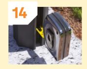
When finishing your fence, the distance between your second last and last post might be less than 1.8m. Simply measure the distance between the two posts, recess edge to recess edge, and cut your boards accordingly.
