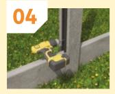
Starting at the bottom, fix the fence post connector to the concrete post with the supplied screws. Don't over-tighten.
