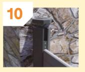
Place a half cap onto the wall post and secure with a rubber mallet.
