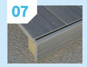
When using an Urban skirt trim across deck board ends, ensure the square edge is in line with the top surface of the Urban deck boards, check there is a 10mm gap between board ends and the vertical edge board.
