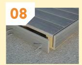
Fix Urban skirt trim underneath the Urban edge board at the joist ends using pilot holes as before. Leave a 50mm gap between ground and the Urban skirt trim to aid airflow. Use two colour coded screws at every joist.
