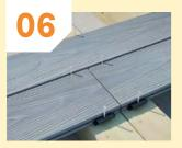
Where board ends meet allow an expansion gap (see expansion table) fit a second supporting noggin and fit a hidden fixing clip at the end of each board.
