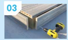
Skirt trims can be used to finish the deck. Fix with two screws at the recommended centres. Drill pilot holes before screwing.
