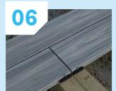
Where board ends meet allow an expansion gap (see expansion table) fit a second supporting noggin and fit a hidden fixing clip at the end of each board.
