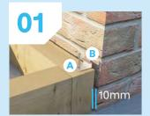
Fix starter clip onto decking joist with screw, allowing first deck board to be installed.
