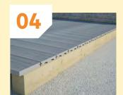
Ensure the Urban deck boards are cut square (see note on conditioning). All board ends should be cut 10mm back from the joist edge when using an Urban skirt trim.
