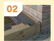
Tilt first deck board so that the leg of the deck locates underneath the lip of the perimeter starter clip.
