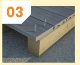
Ensure the colour coded screws are screwed into the pilot holes at 90° with two screws at every joist. Once screwed in place, the head should be flush with the deck surface.
