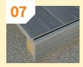
When using an Urban skirt trim across deck board ends, ensure the square edge is in line with the top surface of the Urban deck boards, check there is a 10mm gap between board ends and the vertical edge board.
