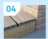
Slide the next deck board into position, locating the hidden fixing clip into its groove. This will set the gap between each deck board. Tighten the hidden fixing clip - but do not over tighten, use a low speed high torque setting on your electric screwdriver. Duplicate this step for every additional board.
