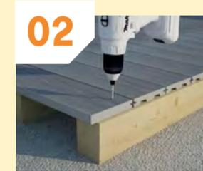
When using the colour coded screws, pre-drill pilot holes first, using a 2mm drill. Ensure pilot holes are no less than 25mm from each edge. Edge boards should overhang the joist by 15mm to cloak the Urban skirting if being used.
