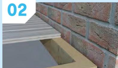
**02** 10mm between the wall and deck board.
