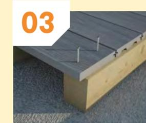
Ensure the colour coded screws are screwed into the pilot holes at 90° with two screws at every joist. Once screwed in place, the head should be flush with the deck surface.
