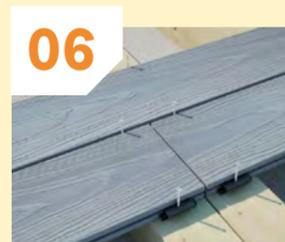
Where board ends meet allow an expansion gap (see expansion table) fit a second supporting noggin and fit a hidden fixing clip at the end of each board.
