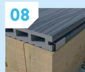
The starter clip is also used as a finishing clip. Install the starter clip to the end of the last joint, slide the deck board between the last clip and the finishing clip.
