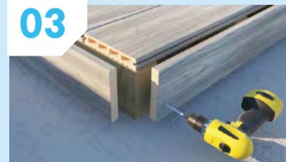
**03** Skirt trims can be used to finish the deck. Fix with two screws at the recommended centres. Drill pilot holes before screwing.
