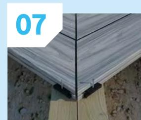
When fitting two boards at 90° ensure a minimum expansion gap of 5mm where the boards meet. Ensure hidden fixing clips are used at both board ends.
