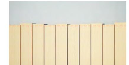
Prior to installation the deck boards, edge boards and edge skirts must be conditioned. Remove from their packaging and lay side by side 24hrs prior to fitting. Then trim to ensure they are all the same length.
