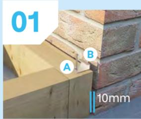
Fix starter clip onto decking joist with screw, allowing first deck board to be installed.
