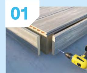
Two pilot holes should be drilled at every joist, leaving a gap of at least 50mm from both the beginning and the end of the trim.
