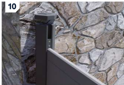
10: Place a half cap onto the wall post and secure with a rubber mallet.
