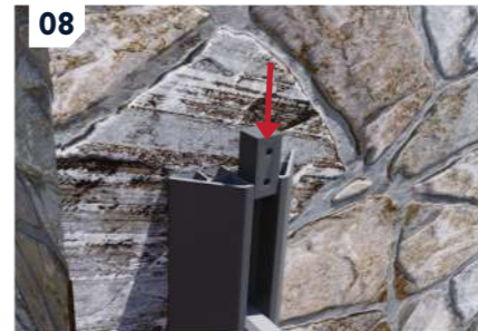
08: Slide a stopper onto each post to sit above the fence finishing rail.
