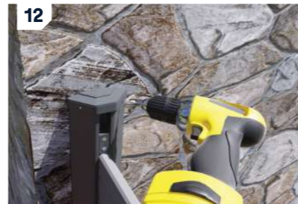
12: Fix the cap to the post with the supplied screws.
