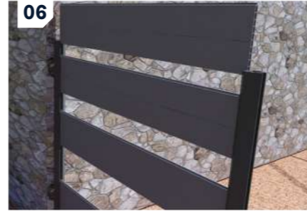
06: Slot in the first fencing board, ensuring it is level before adding the other boards. Each board should sit firmly on the last, similar to tongue and groove.
