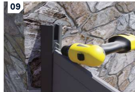
09: Use two screws to fix each stopper into place.
