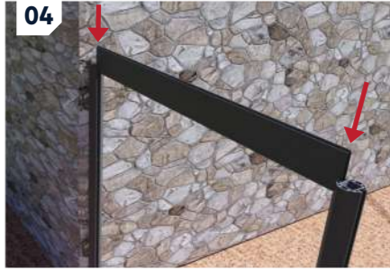
04: Insert the gravel board at the top of both posts and slide it down to the ground.
