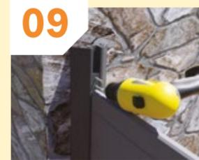
09 Use two screws to fix each stopper into place.
