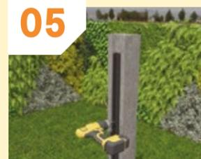
05 Next, fix the top of the fence post connector to the concrete post with the supplied screws.
