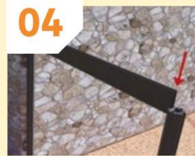
04 Insert the gravel board at the top of both posts and slide it down to the ground.
