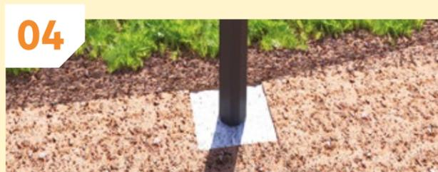
**04** Following the manufacturer's guidelines, fill the hole with concrete, using supports and a spirit level to ensure it stays level on all sides.
