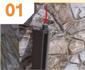
01 Insert the stopper at the top of the wall post, sliding it right to the bottom.
