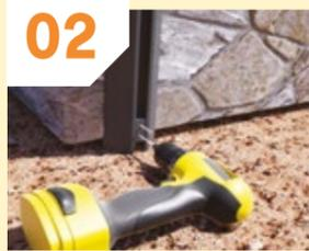
02 Fix the stopper to the wall post with two screws.
