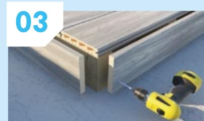
**03** Skirt trims can be used to finish the deck. Fix with two screws at the recommended centres. Drill pilot holes before screwing.
