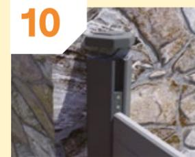
10 Place a half cap onto the wall post and secure with a rubber mallet.
