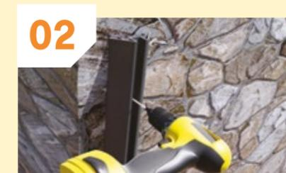
**02** Level the wall post against the wall, keeping it straight and firmly on the ground. Using a 5mm masonry drill bit, drill 50mm pilot hole at the top into the wall.
