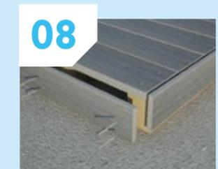
Fix Urban skirt trim underneath the Urban edge board at the joist ends using pilot holes as before. Leave a 50mm gap between ground and the Urban skirt trim to aid airflow. Use two colour coded screws at every joist.
