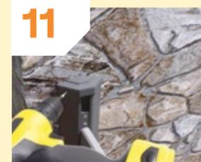
11 Using a 3mm drill bit, drill two pilot holes into the post, using the two predefined holes on the cap as a guide.
