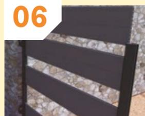
06 Slot in the first fencing board, ensuring it is level before adding the other boards. Each board should sit firmly on the last, similar to tongue and groove.
