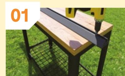
**01** Before fixing the post to the wall, you'll need to pre-drill 5 pilot holes and counter sinks using a 4mm countersink drill bit.
