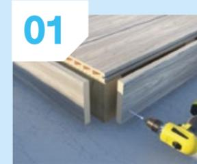
Two pilot holes should be drilled at every joist, leaving a gap of at least 50mm from both the beginning and the end of the trim.
