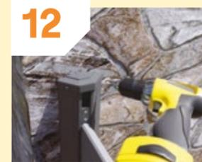
12 Fix the cap to the post with the supplied screws.
