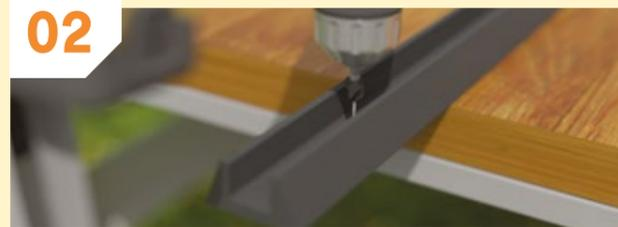
02 Before inserting the fence post connector and fixing it to the concrete post, you'll need to pre-drill 4 pilot holes and counter sinks using a 4mm countersink drill bit.
