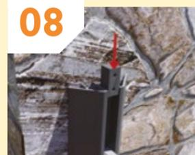
08 Slide a stopper onto each post to sit above the fence finishing rail.
