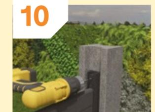
10 Use two supplied screws to fix each stopper into place.
