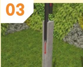
03 Insert the fence post connector into the concrete post recess and use a 4mm masonry drill bit to drill 30mm pilot holes. Ensure the fence post connector is straight before continuing.
