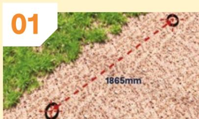
**01** Mark the two post locations 1865 mm apart, centre to centre. This allows the 1.8m fence boards to slot into place when the posts are set.
