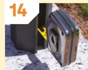
14 When finishing your fence, the distance between your second last and last post might be less than 1.8m. Simply measure the distance between the two posts, recess edge to recess edge, and cut your boards accordingly.
