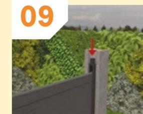
09 Slide a stopper onto each post to sit above the fence finishing rail.
