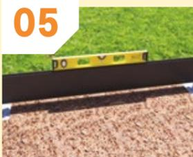
05 Using a spirit level, make sure the board is 100% level
