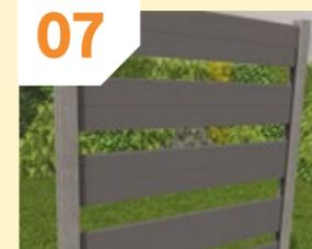
07 Once all fence post connectors are secured, slot 5 fencing boards in one by one, making sure each fits firmly on the bottom board, before stacking on the rest.
