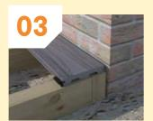
On every joist, position a hidden fixing clip into the groove of the first board and screw into position but do not tighten.
