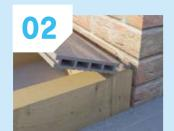
Tilt first deck board so that the leg of the deck locates underneath the lip of the perimeter starter clip.
