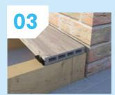
On every joist, position a hidden fixing clip into the groove of the first board and screw into position but do not tighten.
