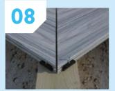
When fitting two boards at 90° ensure a minimum expansion gap of 5mm where the boards meet. Ensure hidden fixing clips are used at both board ends.
