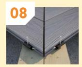
When fitting two boards at 90° ensure a minimum expansion gap of 5mm where the boards meet. Ensure hidden fixing clips are used at both board ends.
