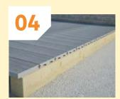
Ensure the Urban deck boards are cut square (see note on conditioning). All board ends should be cut 10mm back from the joist edge when using an Urban skirt trim.
