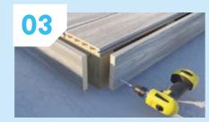
Habitat+ skirt trim can be used to finish the deck on the long end of the boards only. Fix with single screw at 400mm centres. Drill pilot holes before screwing.
