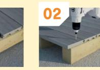
When using the colour matched screws, pre-drill pilot holes first, using a 2mm drill. Ensure pilot holes are no less than 25mm from each edge. Edge boards should overhang the joist by 15mm to cloak the Urban skirting if being used.
