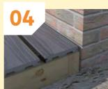
Slide the next deck board into position, locating the hidden fixing clip into its groove. This will set the gap between each deck board. Tighten the hidden fixing clip - but do not over tighten, use a low speed high torque setting on your electric screwdriver.
