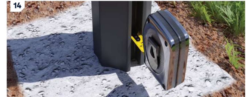
14: When finishing your fence, the distance between your second last and last post might be less than 1.8m.
