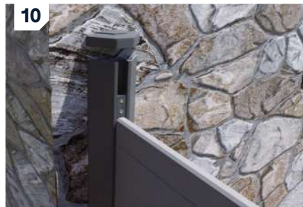
10: Place a half cap onto the wall post and secure with a rubber mallet.
