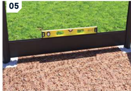
05 Using a spirit level, make sure the board is 100% level.
