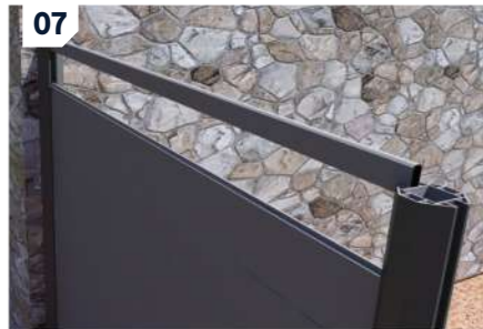
07: Add the fence finishing rail.
